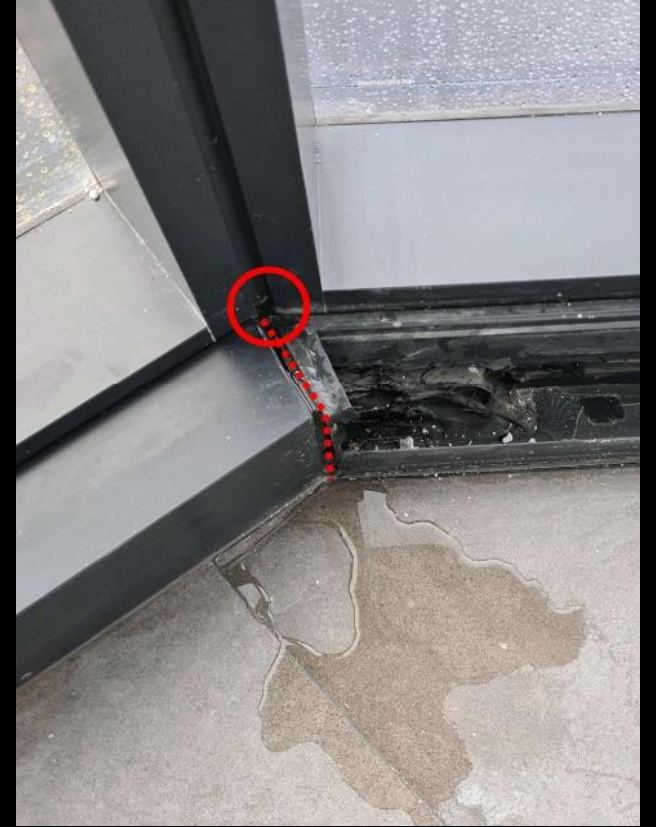
Water ponding on floor
