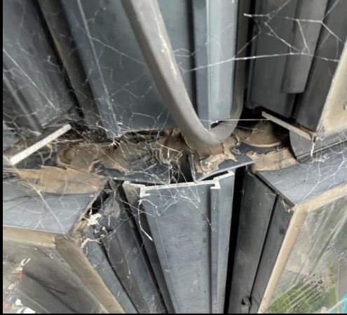
Exposed framing / Missing external sleeves
