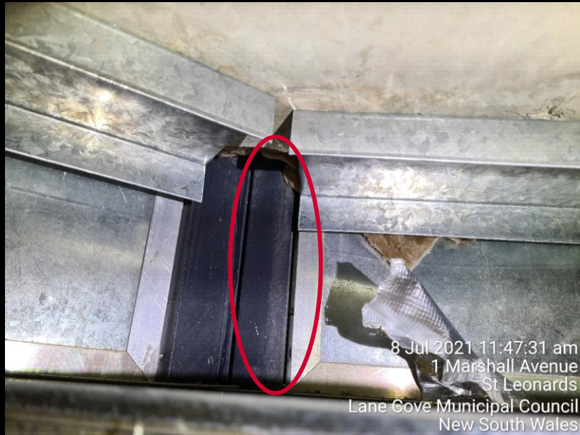
Water Ingress down mullion behind the slab
